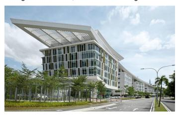
'green', it is really about making people more comfortable and reducing the maintenance cost of the building. So this comes down to the design of the building, like the sun orientation to lessen energy consumption, how do we implement fins to reduce glare and cool the building down," adds Zainal.
